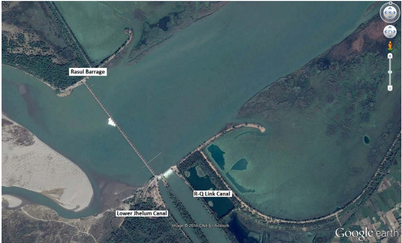
Figure 28 Rasul Barrage showing main barrage and offtake canals
