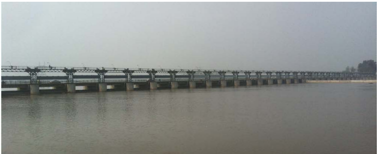
Figure 33 Balloki Barrage showing main barrage
