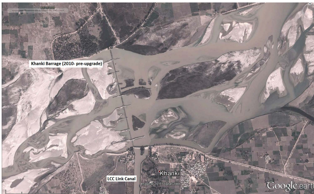
Figure 26 Khanki Barrage showing main barrage and offtake canal
