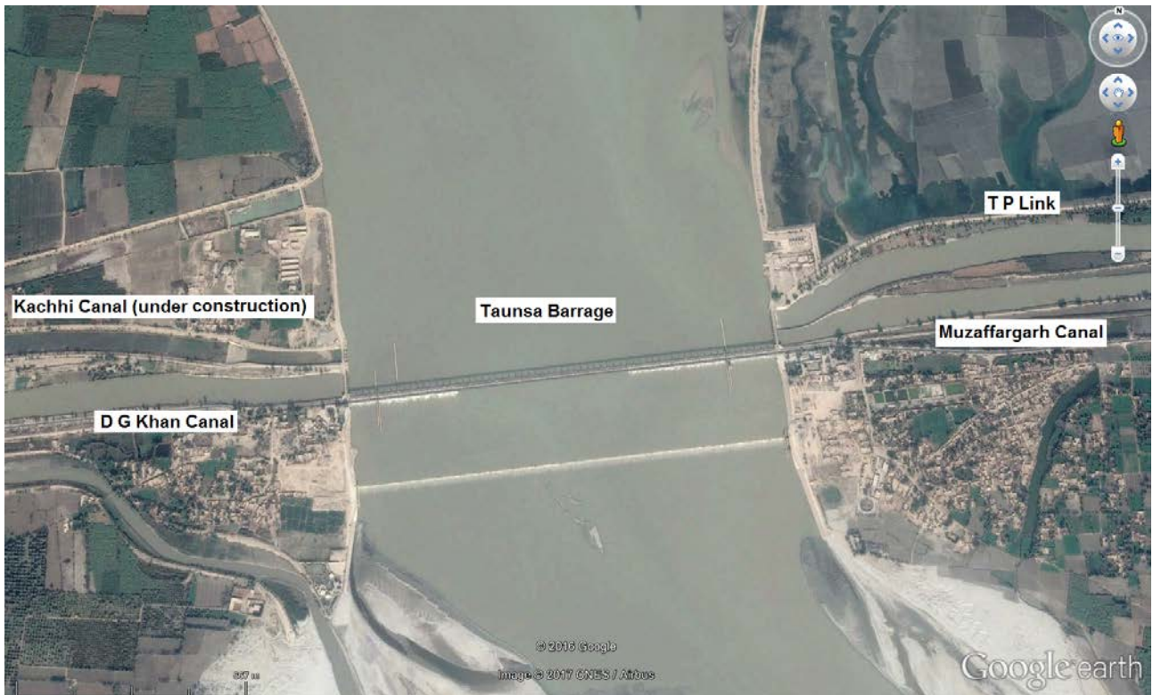
Figure 47 Taunsa Barrage showing main barrage and offtakes
