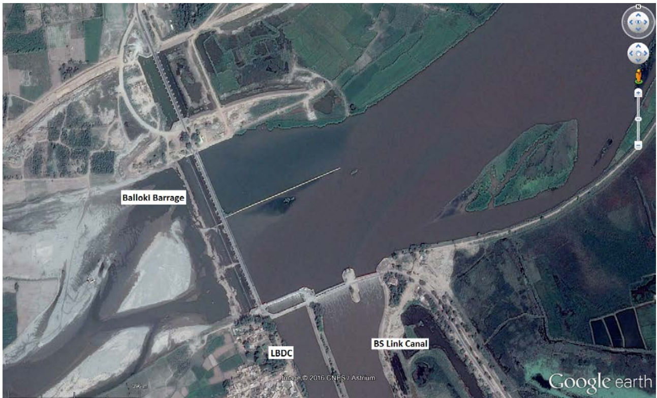
Figure 32 Balloki Barrage showing main barrage and offtake canals
