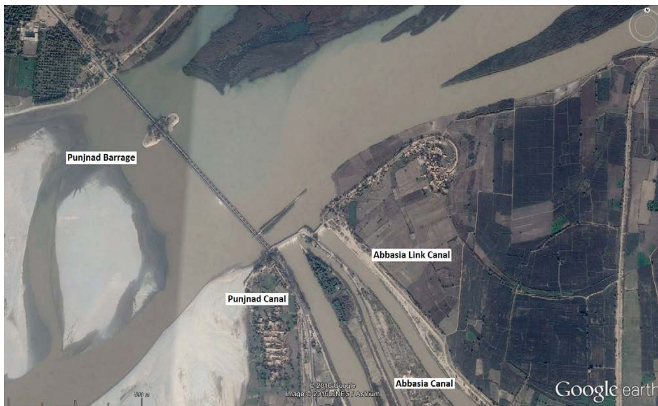
Figure 39 Punjnad Barrage showing main barrage and offtake canals
