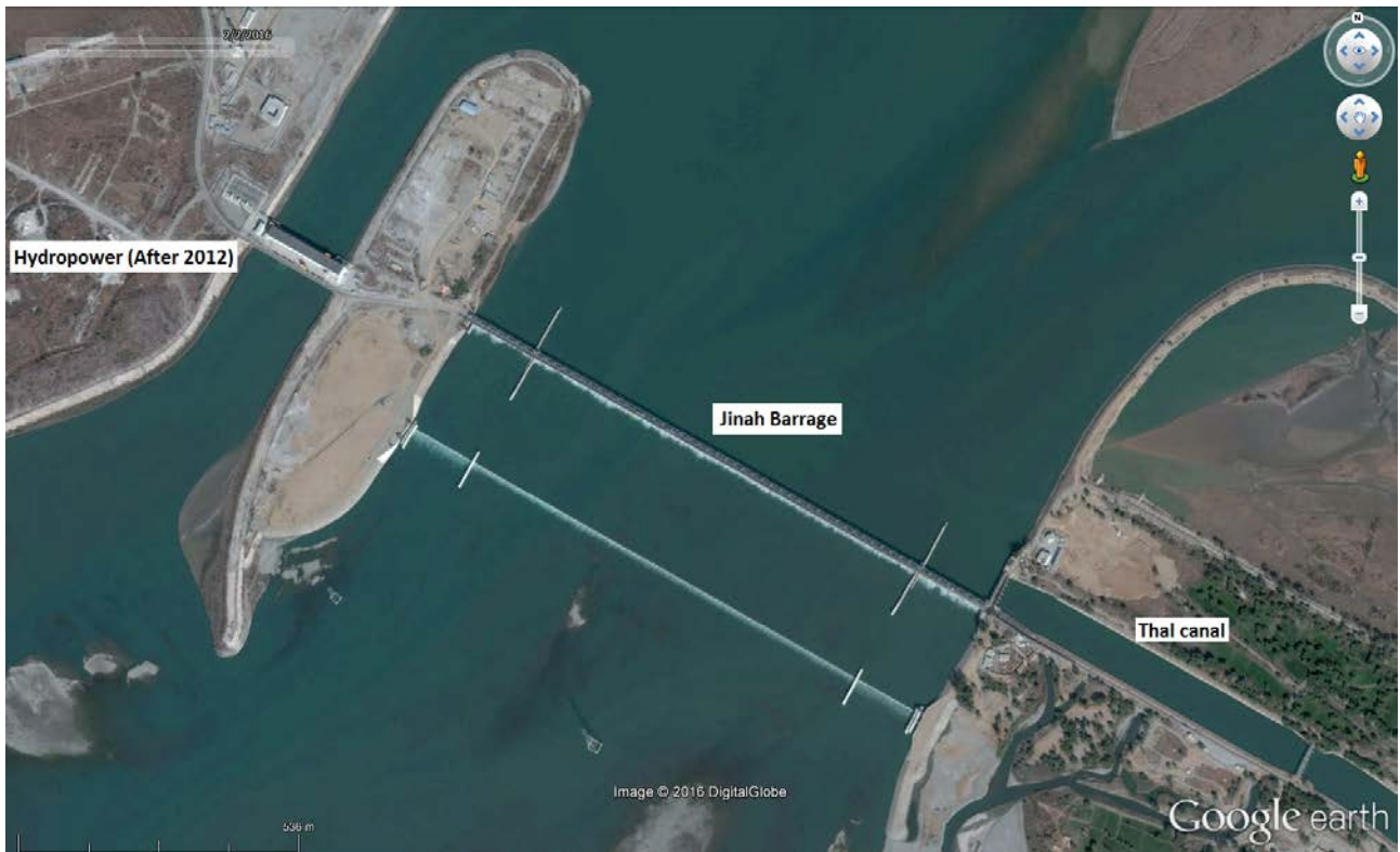
Figure 45 Jinah Barrage showing main barrage 2012 hydropower and Thal Canal offtake
