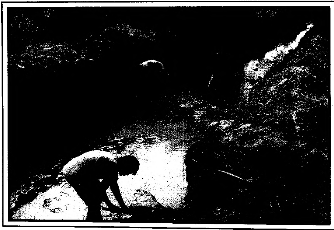
Manual desilting of Chahu Minor during the rotational closure (August 1997).
