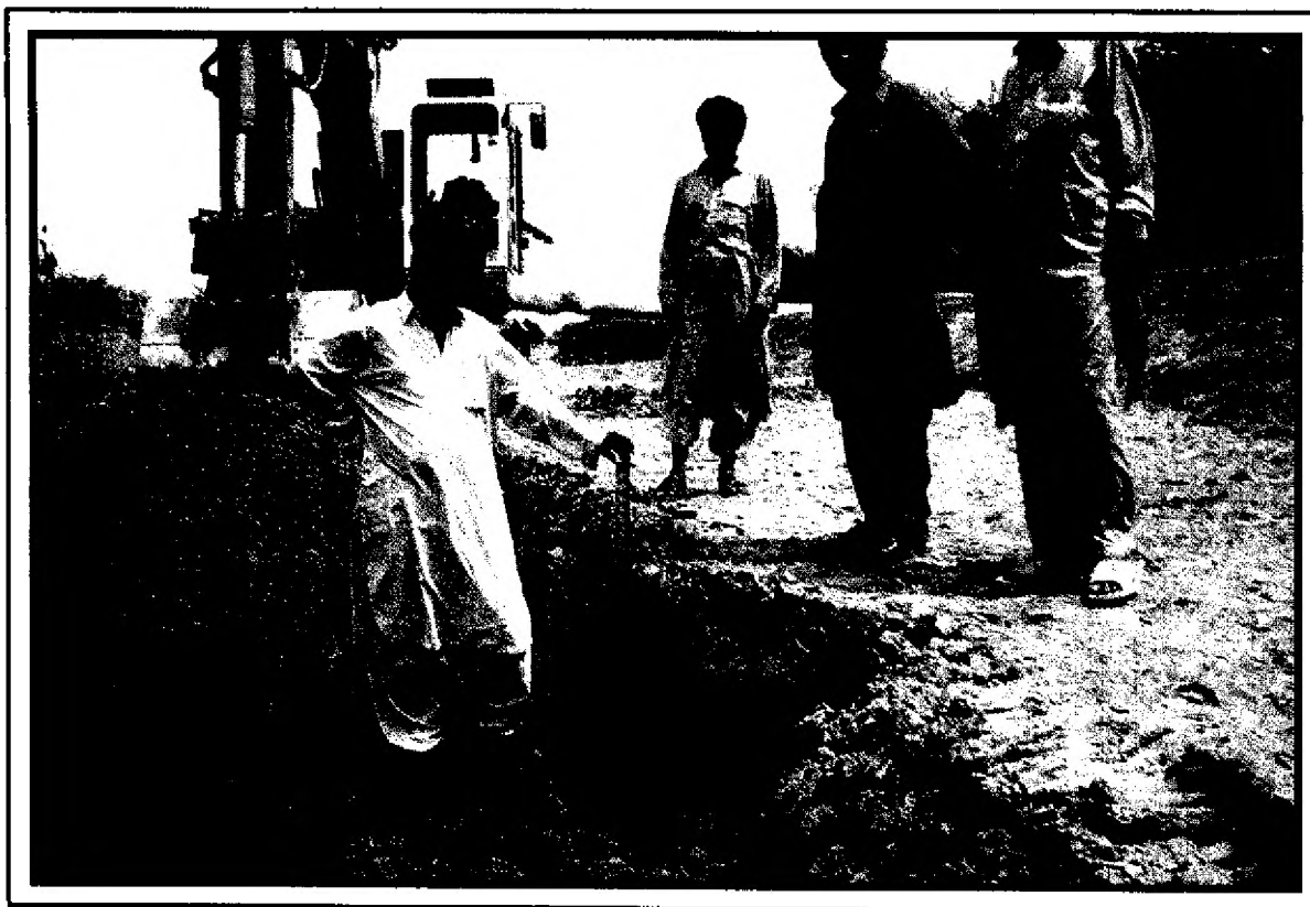
Desilting by machine in Digri Sub-division (March 1997).
