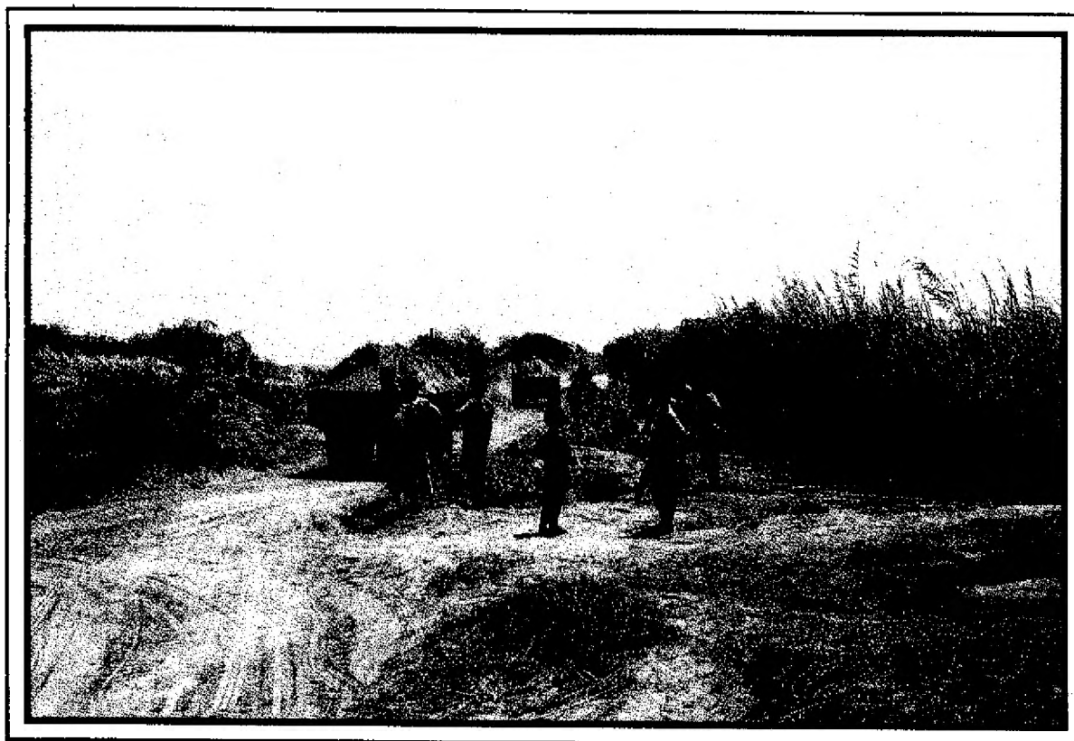
Removal of sand heaps after the desilting of Jarwari (July 1997)
