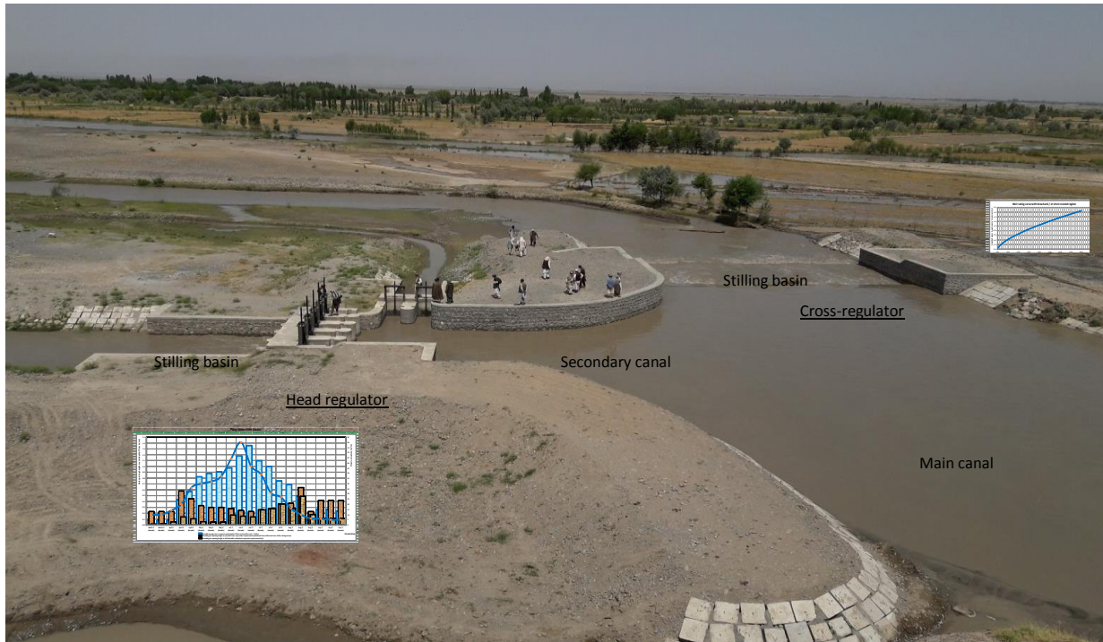
Figure 2.4: bird view of Selaba head work with ungated cross-regulator and rating curve on the right and gated head regulator with canal hydrograph and corresponding gate(s) openings on the left (Yatim Tepa canal)
